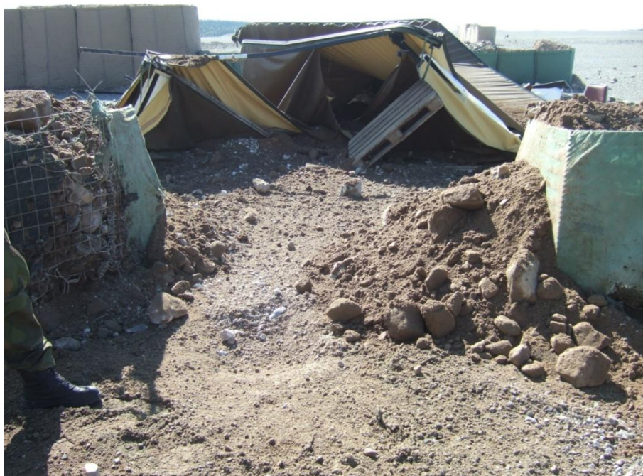
Figure 2.26 MIL 3 wall with local soil after detonation of a 155 mm grenade (test 1.12)
