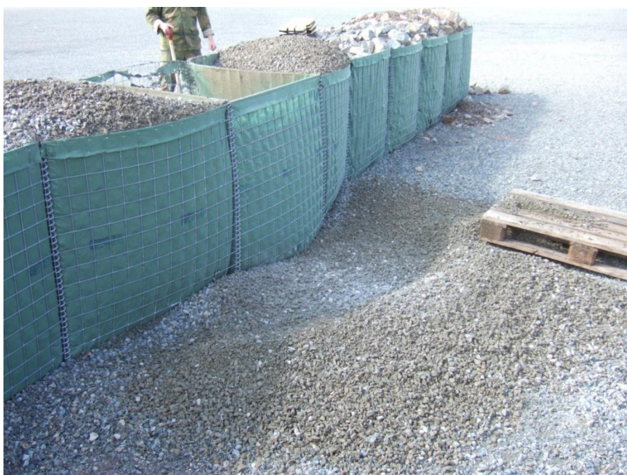
Figure 2.15 Back side of MIL 3 wall with gravel after detonation of 7.5 kg TNT (test 1.8)
