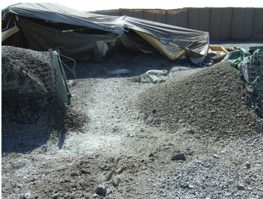
Figure 2.27 MIL 3 wall with gravel after detonation of a 155 mm grenade (test 1.13)
