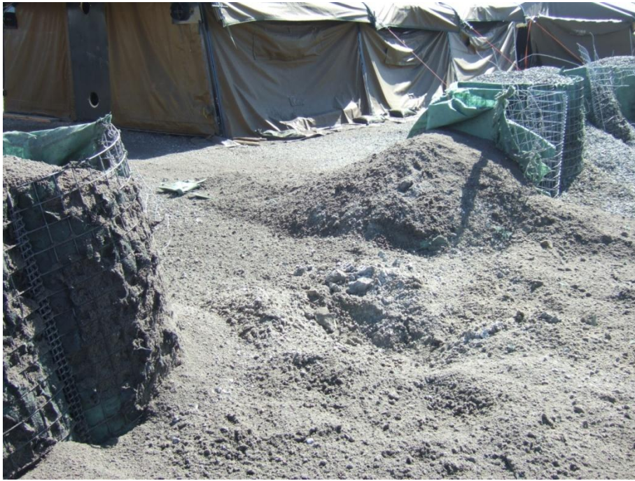
Figure 2.24 MIL 3 wall with sand after detonation of a 155 mm grenade (test 1.11)
