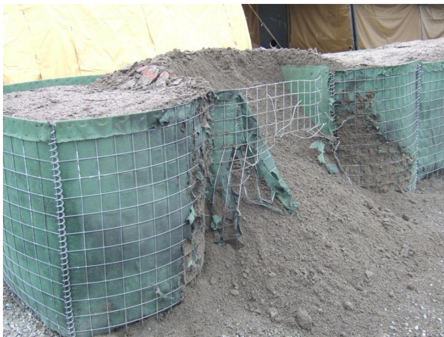
Figure 2.8 Front side of MIL 3 wall with sand after detonation of 3.5 kg TNT (test 1.1)
