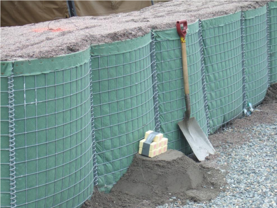
Figure 2.3 Setup of test 1.1 with 3.5 kg TNT at a MIL 3 wall with sand
