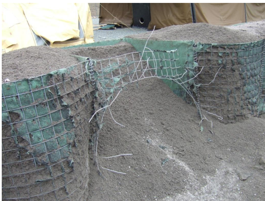
Figure 2.9 Front side of MIL 3 wall with sand after detonation of 7.5 kg TNT (test 1.2)
