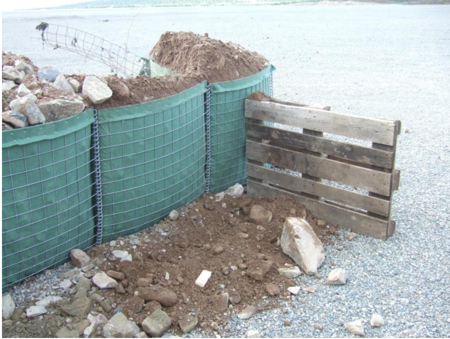
Figure 2.20 Back side of MIL 3 wall with local soil after detonation of 3.5 kg TNT (test 1.10)
