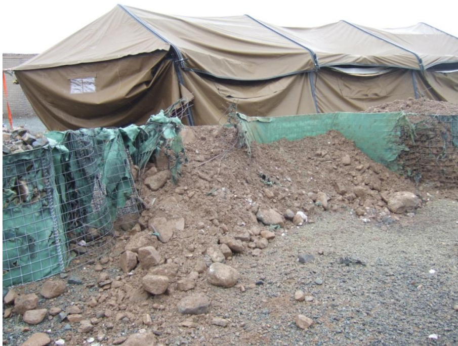
Figure 2.22 Front side of MIL 3 wall with local soil after detonation of 7.5 kg TNT (test 1.7)
