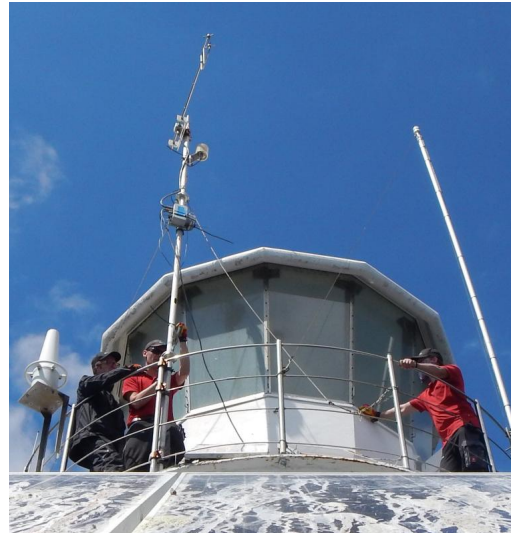
Figure 3: Permanent installation on Roman Rock Lighthouse (left side: total view). Meteorological sensors have been installed on top of the lighthouse (right side), while a BLS 900 emitter was installed at the base of it.
