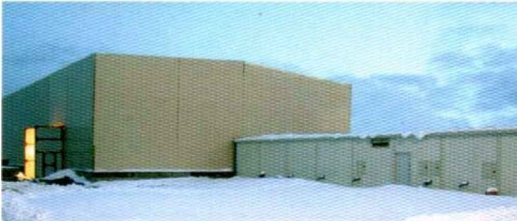
Picture 4. The outside picture of the integrated radioactive waste treatment and storage installation (PPP-RAO) at FSUE “10 SRP” as it nears completion in December 2003; the storage pad with weather enclosure are on the left and the MPF is to the right of this picture.
