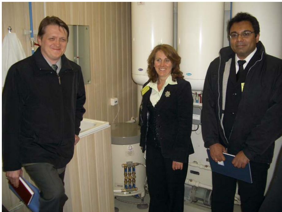
Picture 6. Presentation of the water radiation activity sensor to U.S. and Norwegian representatives 14 June 2005, installed to monitor water discharges from the PPP-RAO facility.
