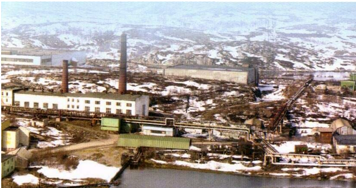
Picture 1. The Federal State Unitary Enterprise 10 th Ship Repair Plant of the Russian Ministry of Defence in Polyarny (FSUE “10 SRP”).
